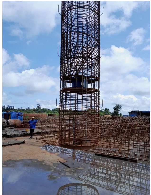
Reinforcing cage, O-cell® and instrumentation prepared by Julius Berger Nigeria PLC
